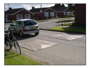
Alternatively, speed cushions could be considered in place of full-width road humps. These are generally more comfortable for cyclists to negotiate than fullwidth road humps since they can usually avoid riding over the cushions. Usually placed in rows of two or more units across the road, cushions are also sometimes used singly where physical features, such as central traffic islands, limit the usable width to one lane.
