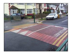
Flat-topped hump using preformed sinusoidal units
